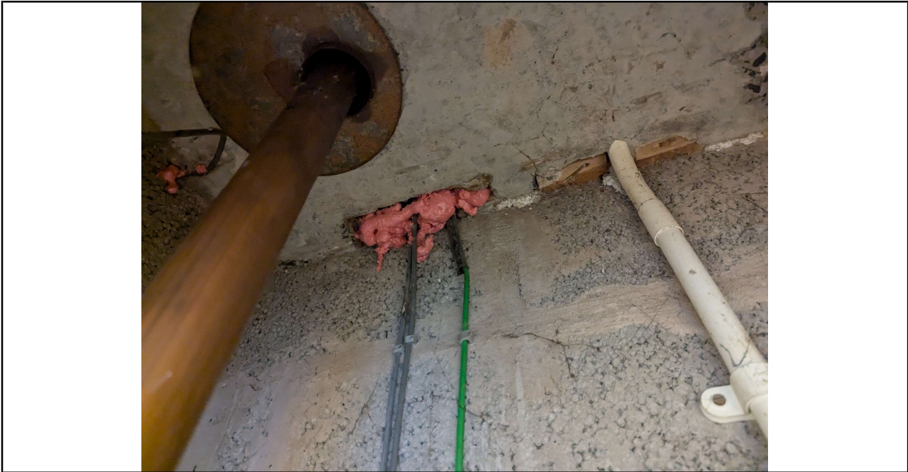
Photo No. 1 Example of Pink Foam in all Meter cupboards
